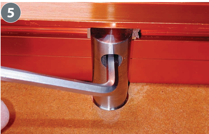
05. Tighten the hex socket bolts firmly.
