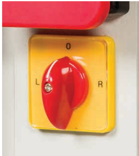
Reversing selector switch
